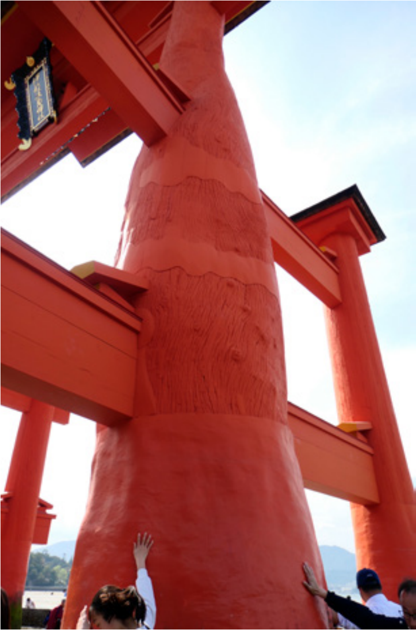
Close-up of the Great Torii at low tide when you can walk out to the gate, photograph, and revere it, noting its vermilion pillars, cypress bark roof, and copper plates, all newly restored from 2019 to 2022 to improve earthquake resistance.
